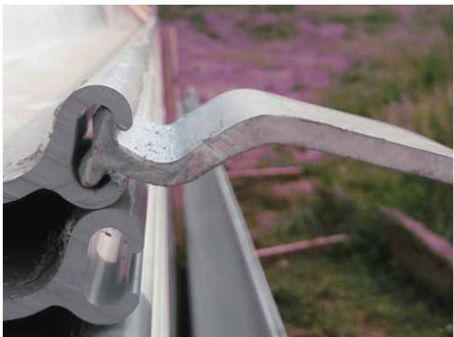
Inspect the interlock. Use a small brush to fill in, smooth or thin any spots if necessary. Watch the thickness of the P-201 Too much P-201 will inhibit the driving process.
