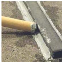
Place a nail or screw every 12~14 inches if concrete must be placed immediately.
