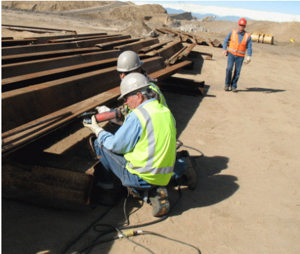
CLEANING INTERLOCKS WITH DRILL MOUNTED WIRE BRUSH
