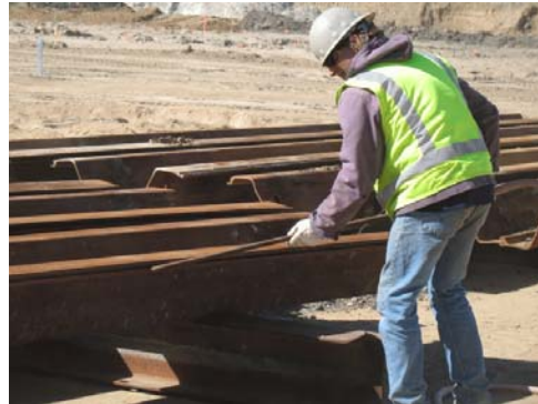
REMOVE DEBRIS BY AIR AFTER CLEANING INTERLOCKS
