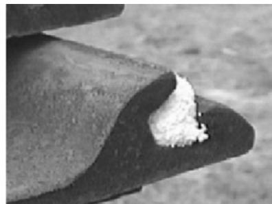
Use urethane foam or similar material to dam ends of interlock.
